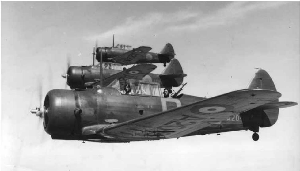
**CAC Wirraways in flight. The Lewis machine gun in the rear cockpit was of little use against an attacking Zero fighter**
