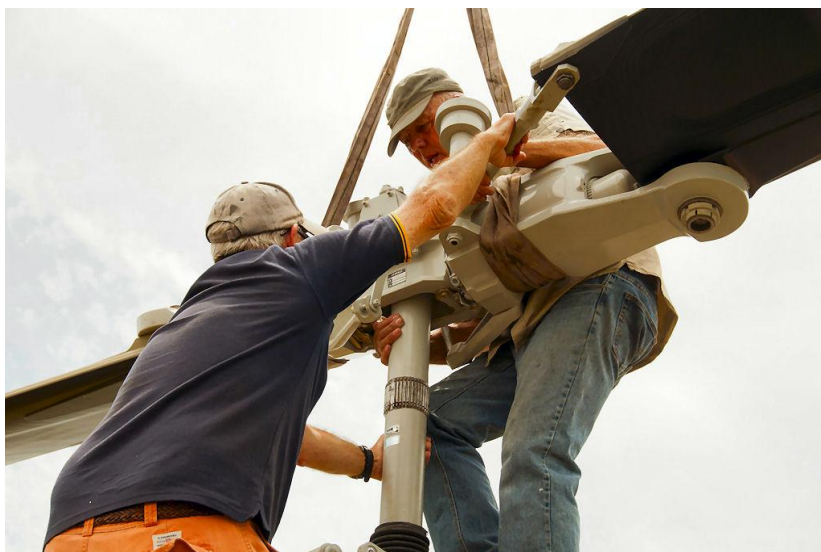
Lining up the splines
