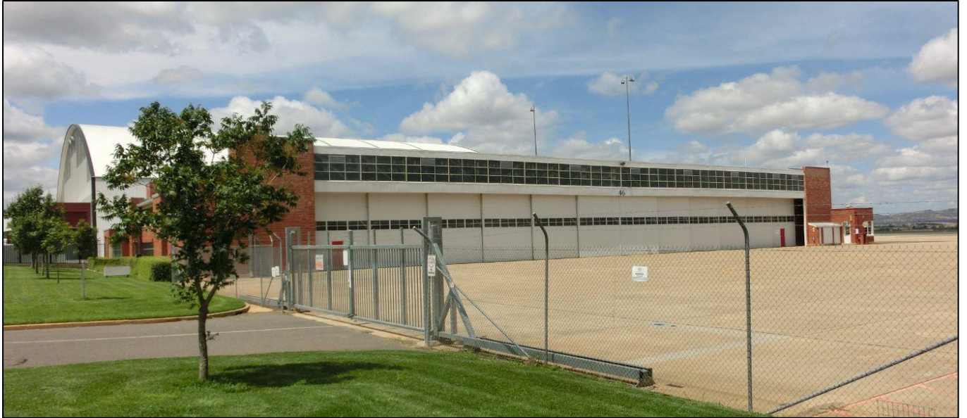
“Old” 5 Squadron Hangar
