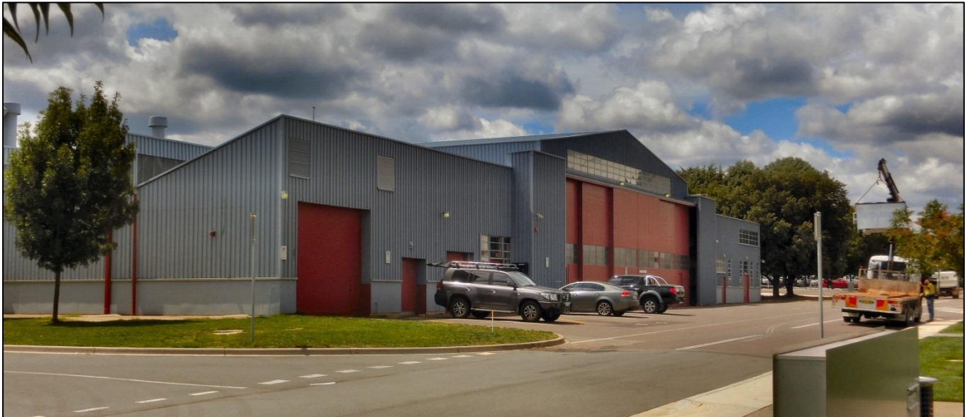
Old Maintenance Hangar
