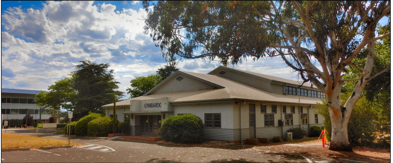
The old ASCO shop and theatre. Today this building is used as a child minding centre for kids of the people who work on the base.
