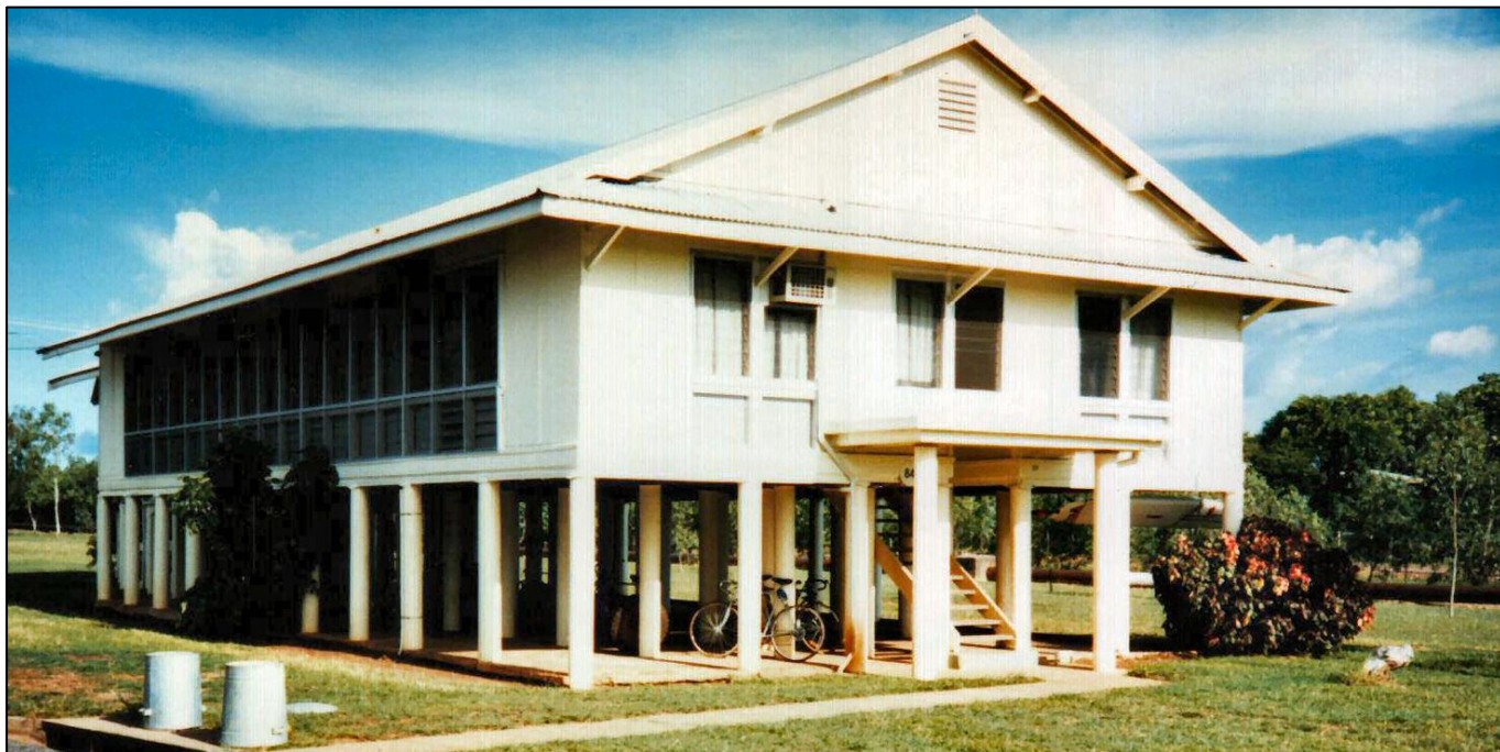
Airman's Accommodation block.
