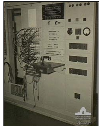
Werribee Receiving Station, antenna switching panel
