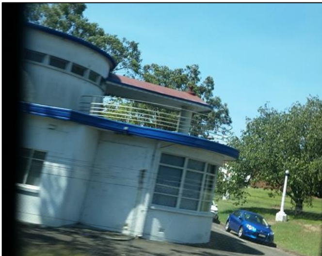
The old Switchie room, Glenbrook, way back!!
