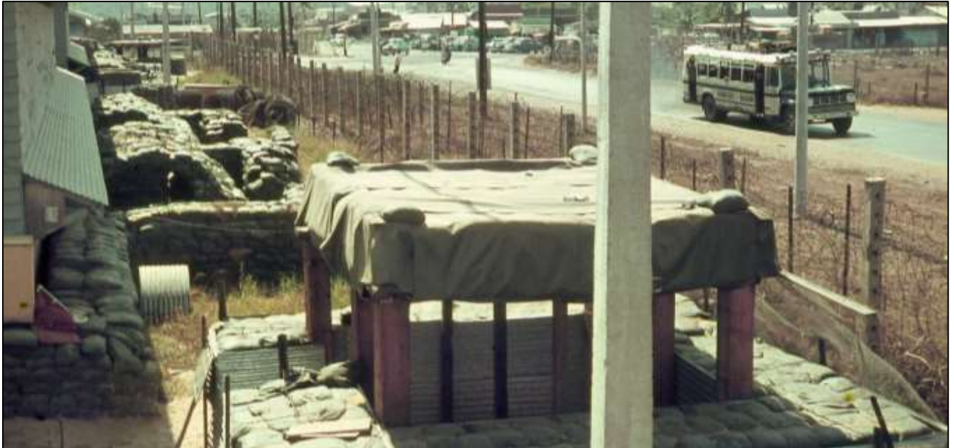
Looking towards the entrance to the Vung Tau airfield from the airmen's dongas. The road heading off to the right from the intersection at the top of the pic headed off into town.
