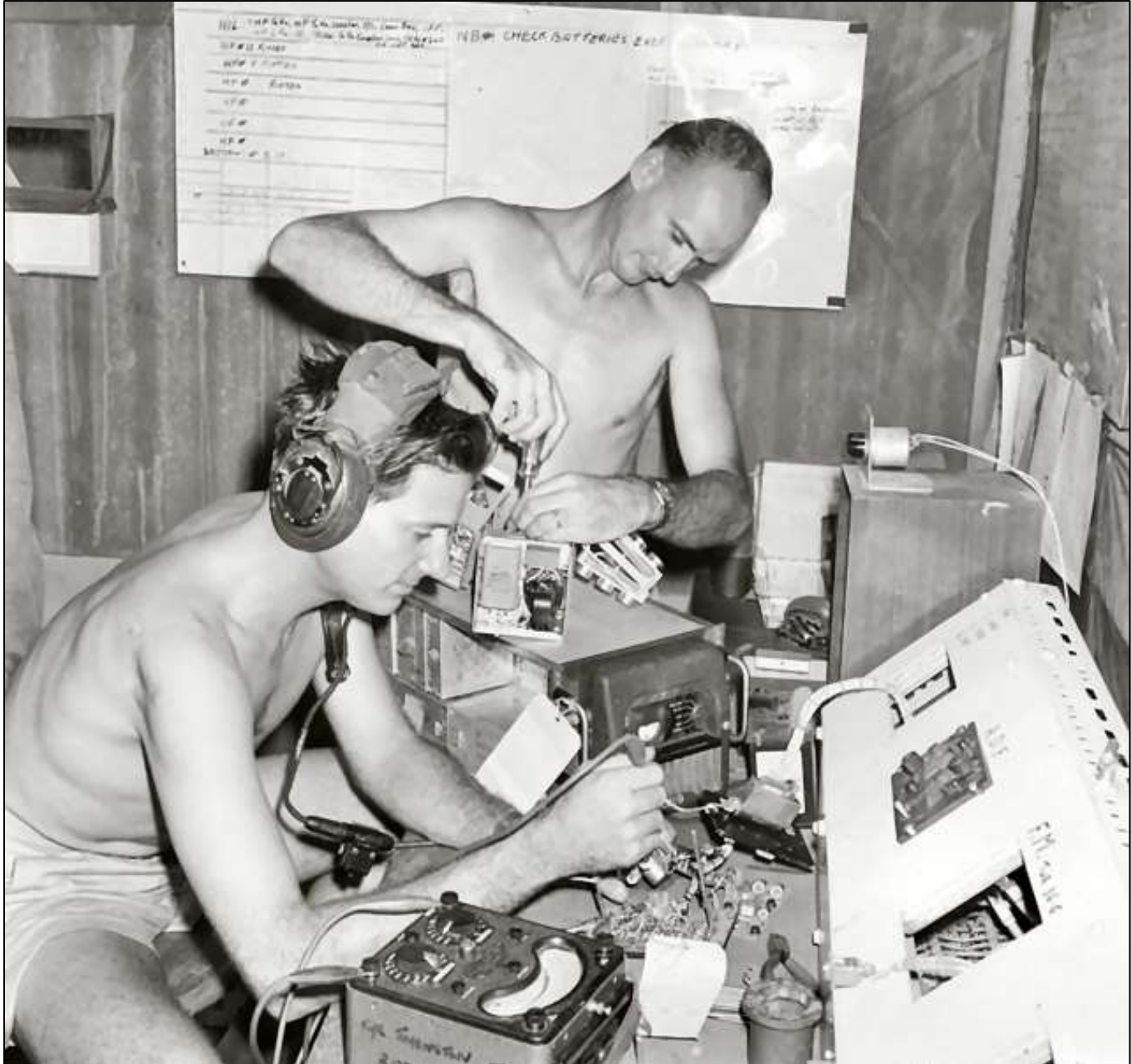
Jack Bennett (seated) and Bruce Barter working on the 618T and antenna coupler.
