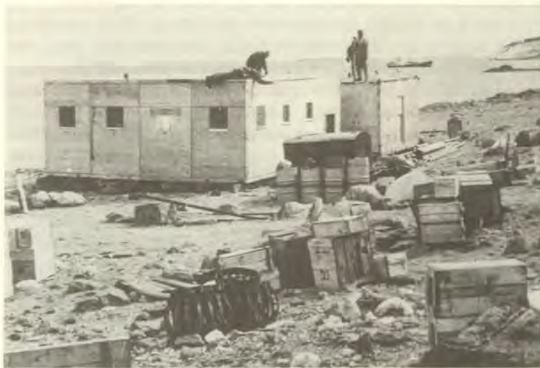
Construction of the base at Davis. (RAAF Official)
