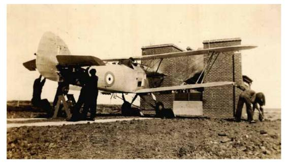
1936: Hawker Demon test firing its machine guns at the stop butts—the engine needs to run to check the interrupter gear (RAAF Museum)
