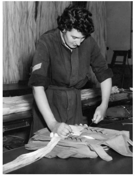
1942: packing rigging lines for a parachute (State Library of Victoria)
