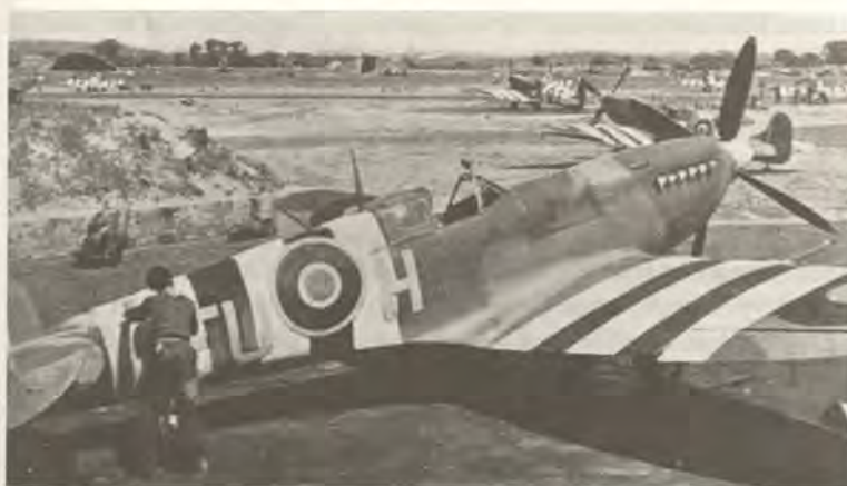
453's Spitfire IXB MK355 FU-H has D-Day invasion stripe identification markings applied at Ford on 4 June 1944.
