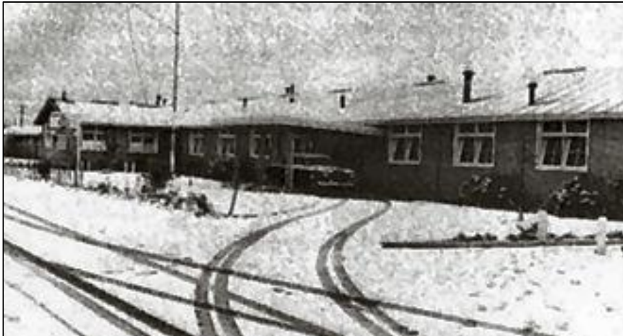
A wintry Entrance to the HQ Building.
