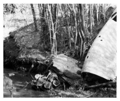
Another view of A19-208 in Coirwong Creek, showing (left) a Hercules engine under the starboard wing root and (right) the fuselage mid-section sloping up the bamboo covered bank
