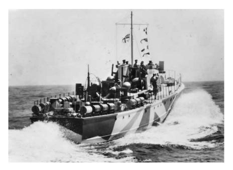
RAN Fairmile motor launch ML 814 at speed. The depth charges seen aft were not carried on Operation Adder
