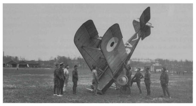
A good landing is one you can walk away from — only minor damage was sustained by Captain H G Forrest's SE-5A C9539 from this mishap at Savy in March 1918, and the aircraft was repaired, eventually to be withdrawn from service as "war worn" in June 1918. AWM E1882
