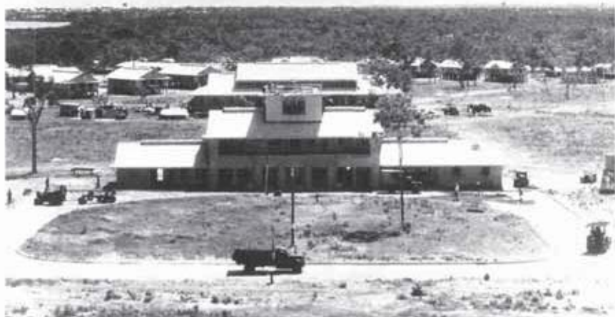
Station Headquarters Darwin under construction, December 1940
