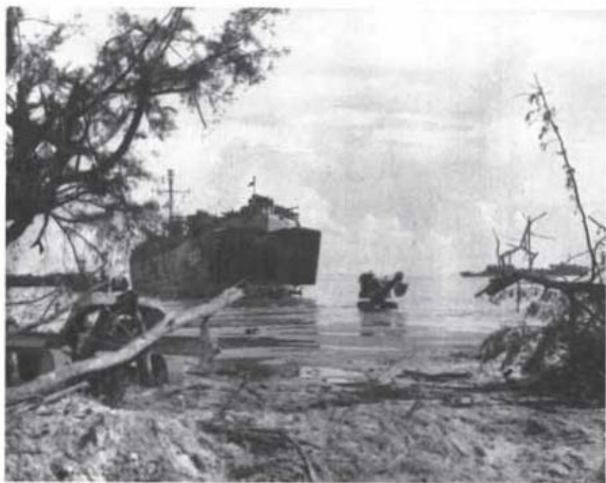
Airfield construction equipment disembarked from an LST, Borneo, 1945
