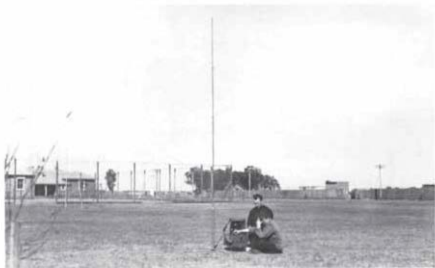
Portable wireless equipment in use at Richmond, August 1932
