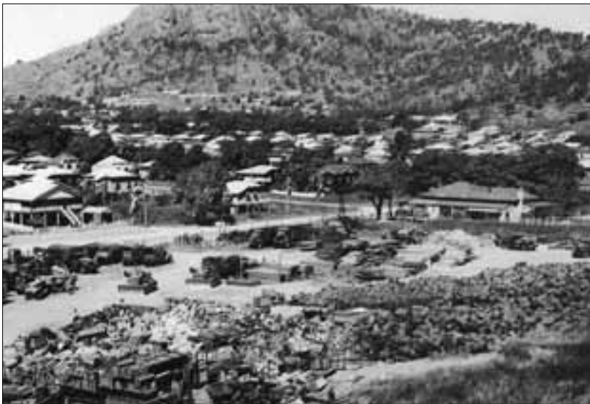
Townsville, 1942 War stores dumped on the beach
