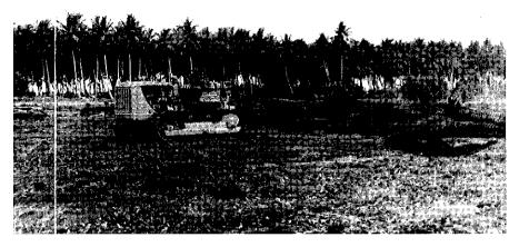
A major problem to be overcome before construction of the main airstrip at Cocos Island was the removal of wartime pierced steel planking. This was overcome by using a D-7 or D-8 tractor to cut it into 50 metre squares so that it could be rolled for ease of handling. (RAAF Museum)
