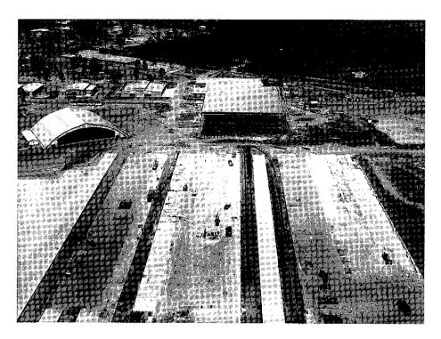
5ACS Detachment 'C' extended and reconstructed the hardstanding at RAAF Base Amberley between June 1967 and September 1969. This photograph shows progress as at February 1968. (RAAF)
