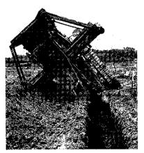
A Barber-C ditcher bogged on the Tarakan airstrip. An example of the waterlogged conditions under which 1ACS strived to build an airstrip. (L. Bloom)
