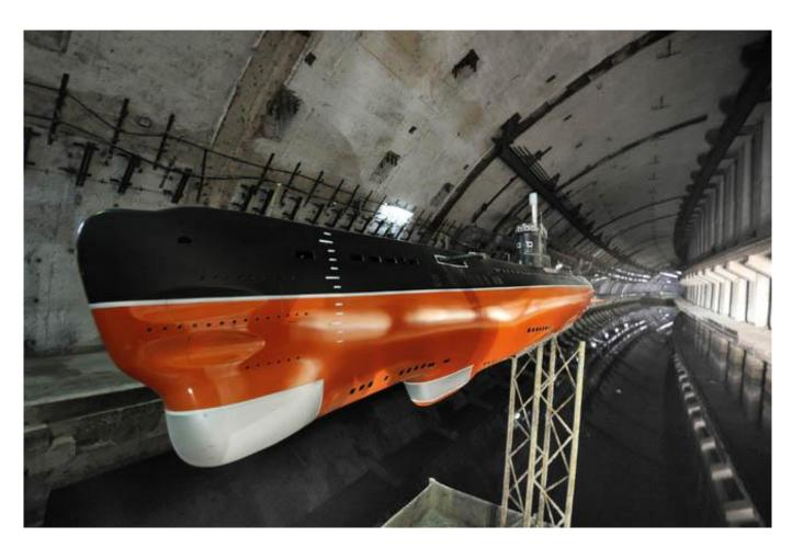
It contained a dry dock so large that it was capable of holding a 300 foot (91 meters) long submarine. Beside the dry dock was the huge submarine channel, with space for six such subs end to end. Curved to deflect any blast inside the base, the channel is lined with steel
