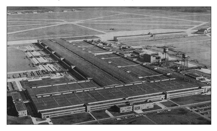
As big and as modern as the other plants were, they were dwarfed by the vast new purpose-built factory constructed by the Ford Motor Company at Willow Run near Detroit, Michigan. Ford broke ground on Willow Run in the spring of 1941, with the first plane coming off the line in October 1942. It had the largest assembly line in the world (3,500,000 ft²/330,000 m²). At its
