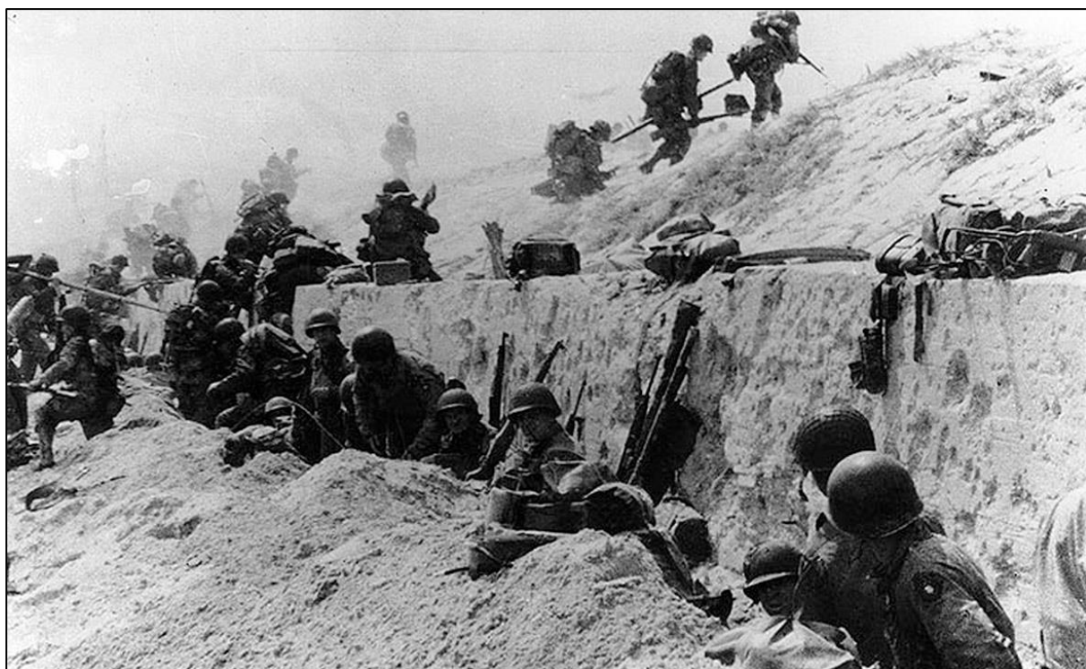
June 6, 1944: US Army soldiers of the 8th Infantry Regiment, 4th Infantry Division, move out over the seawall on Utah Beach after coming ashore in front of a concrete wall near La Madeleine, France.
