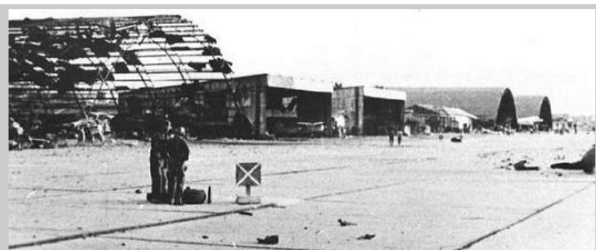
Above: The scene that confronted the Hercules crew at Pochentong. Communist Sappers had effectively destroyed every aircraft at the airport, along with numerous hangars and other infrastructure.
