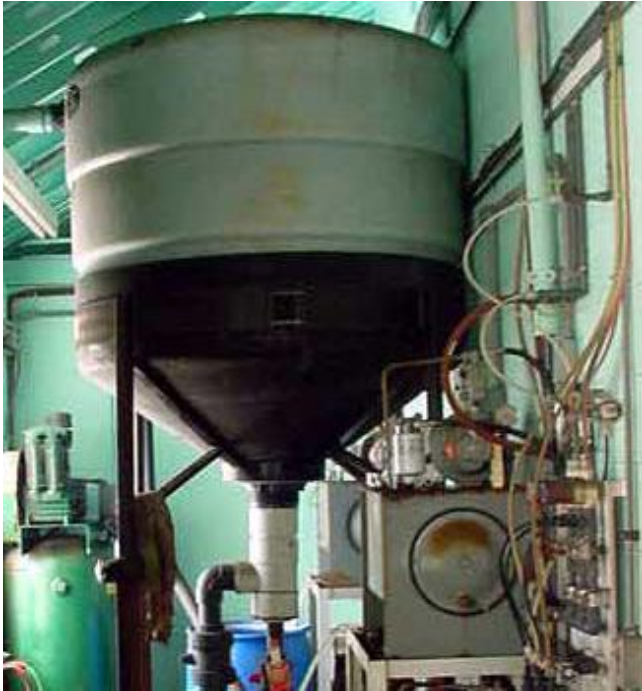
The pressure tank for a high-pressure washer.
