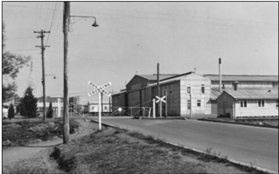
The railway line as it was back in 1957. This was originally the entrance to operational area of the Base, the road, being Newton Rd, leads back to the old Guard Room.
