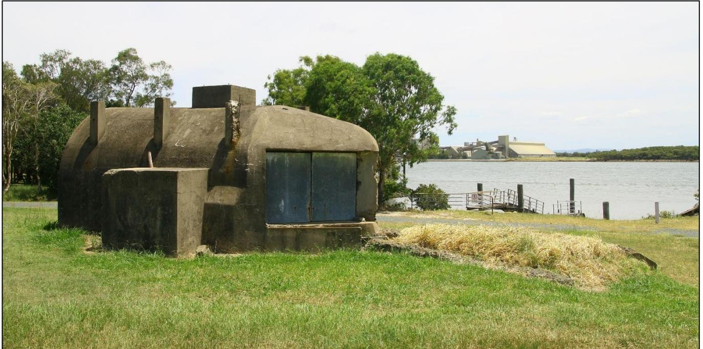
The search-light bunker. This static installation consisted of the light within a concrete emplacement near the river bank closer to the jetty than the Fort. The "Clark Chapman" searchlight could also be mounted on a light railway carriage and was then able to be moved to the best position for its use. The light consumed 50 amps at 75 volts DC.
