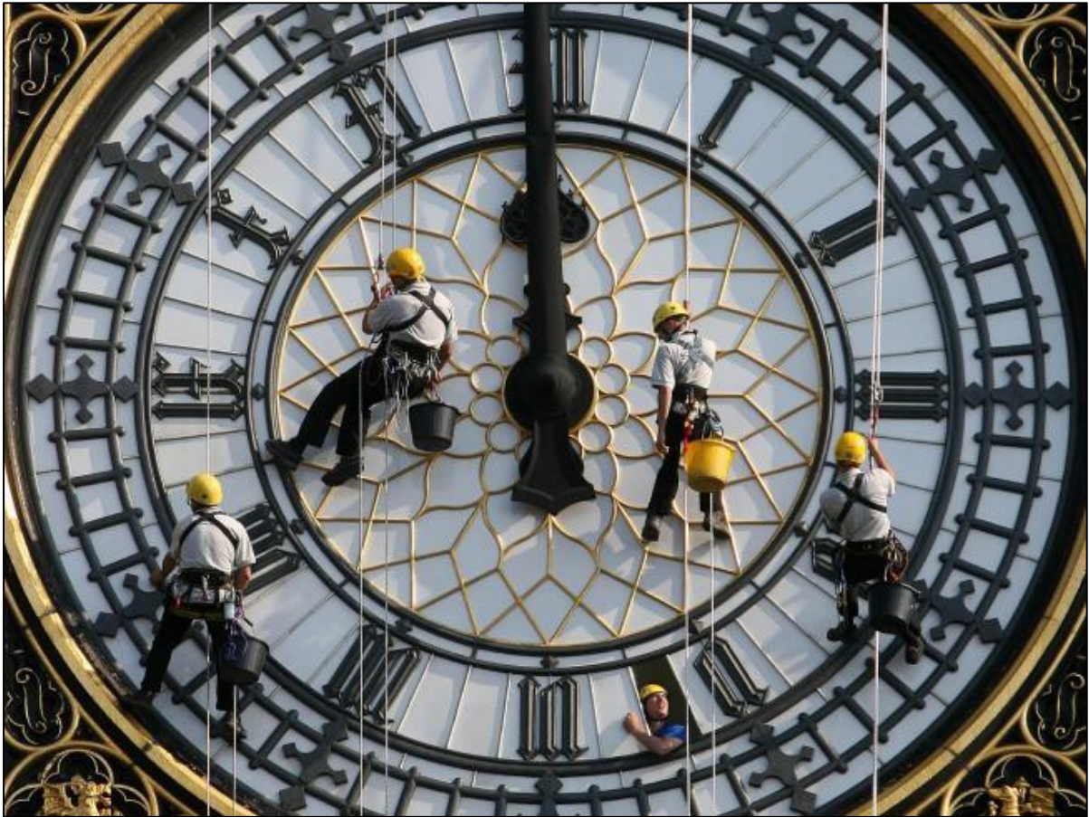
Workers suspended by ropes carry out cleaning and maintenance work on the clock face of Big Ben.
