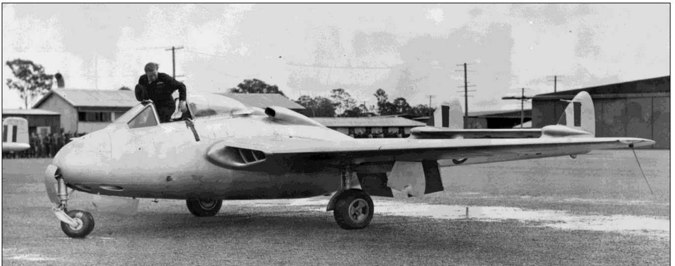
Vampire Mk 30 with elephant ears on top of the engine.
