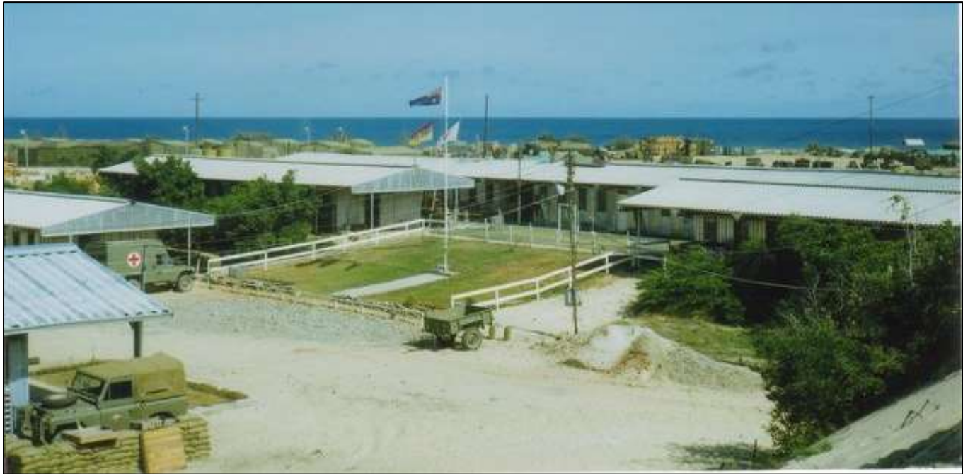
1st Australian Field Hospital, Back Beach, Vung Tau.
