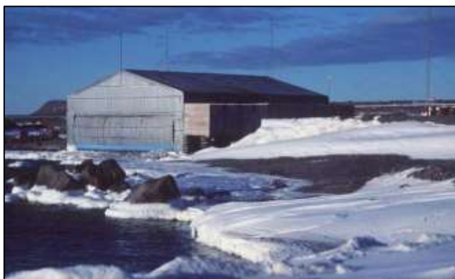
RAAF Mawson Hangar on the end of East Arm, 1983
