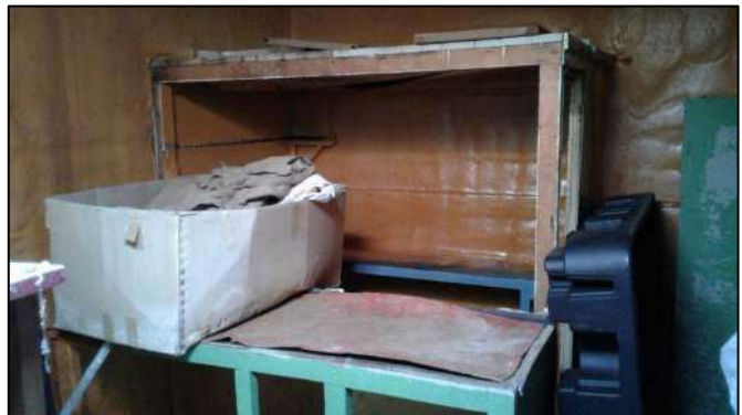
Radio Transceiver rack, south west corner in the radio room.
