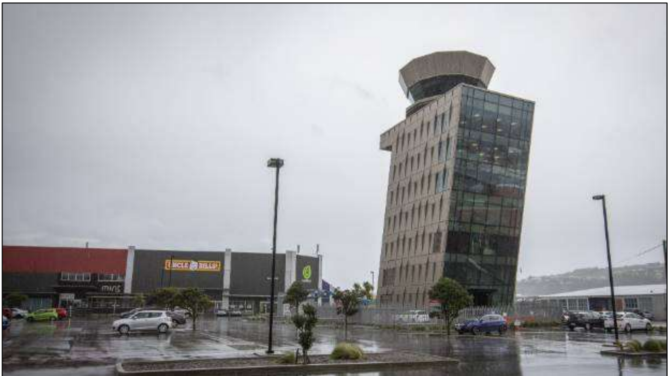
The New Tower building, "The leaning tower of Wellington?".
