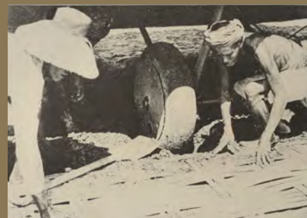
BELOW Bamboo matting formed an improvised runway over mud at Surabaya.
