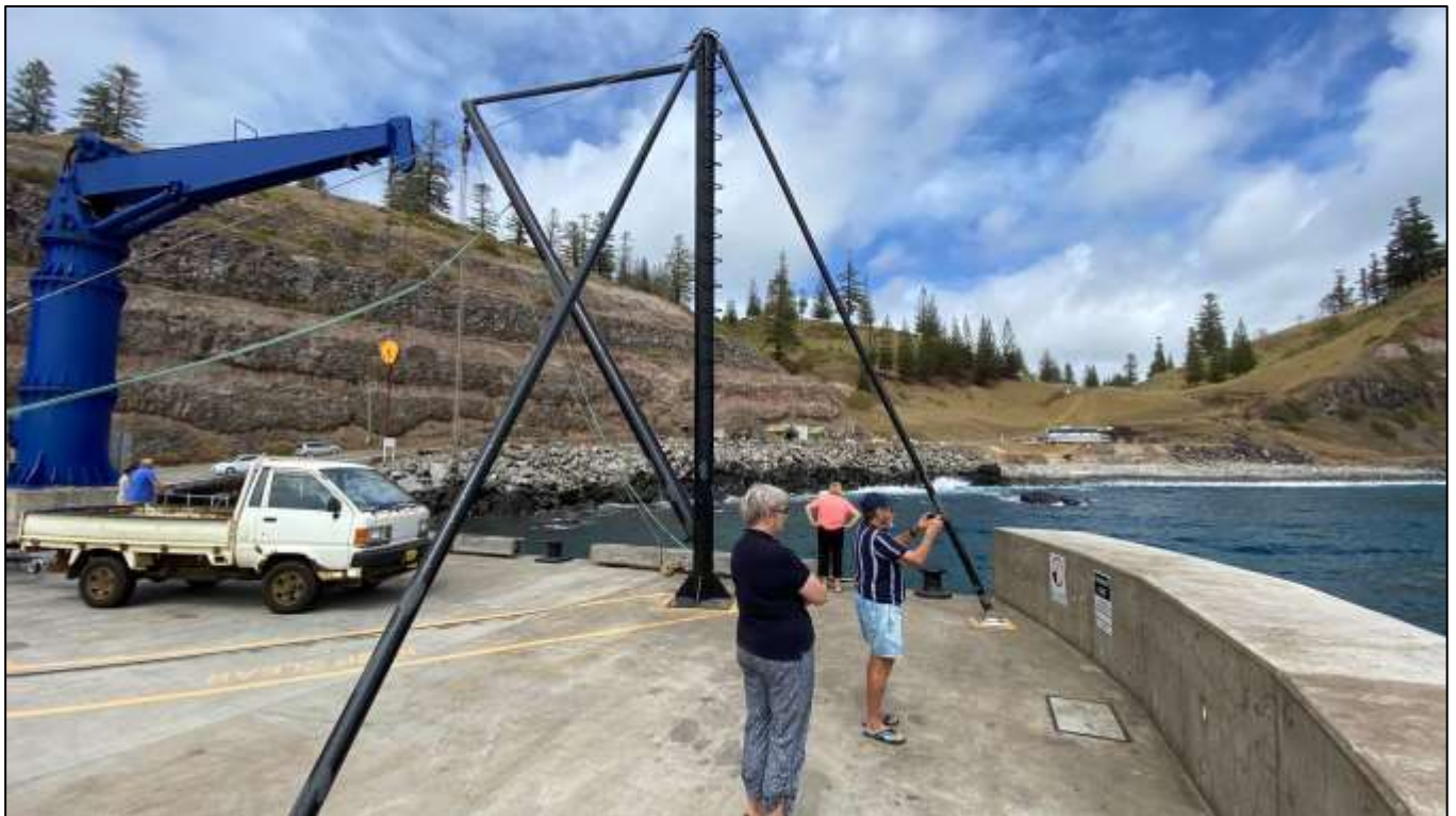
The jetty where all goods brought onto the Island are off loaded.
