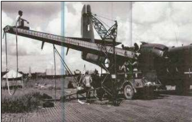
Loaned US Army wing being fitted.
