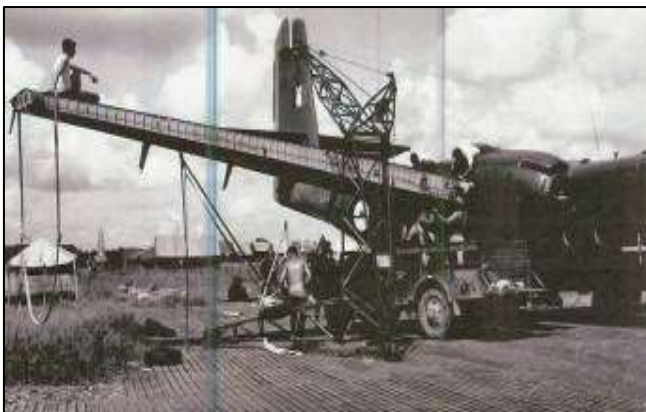
Loaned US Army wing being fitted.
