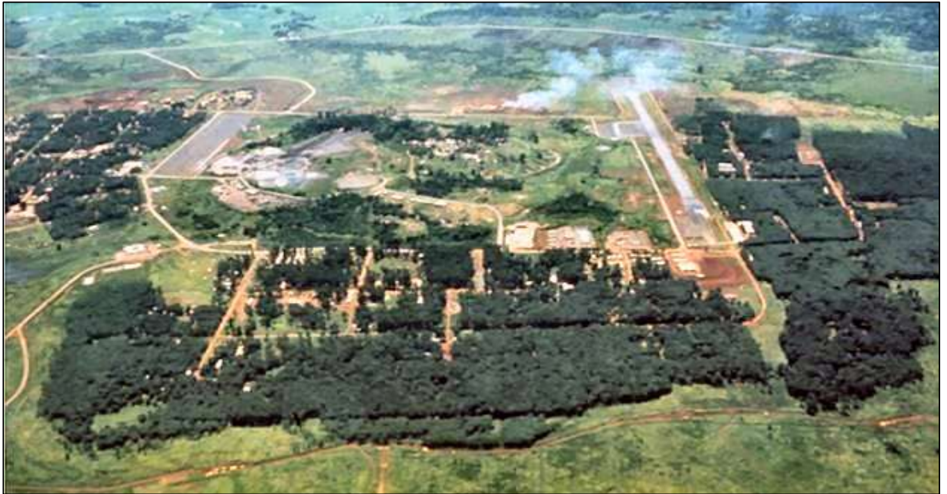
Nui Dat, with Luscombe Airfield on the right. Luscombe Airfield was named after Lt Bryan Taylor Luscombe, the first Army pilot killed in the Korean War. Work on the airstrip was started soon after the Australians arrived at Nui Dat in June 1966.
