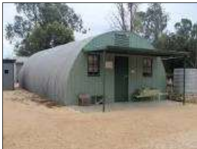
A Nissen Hut similar to Hut 230
