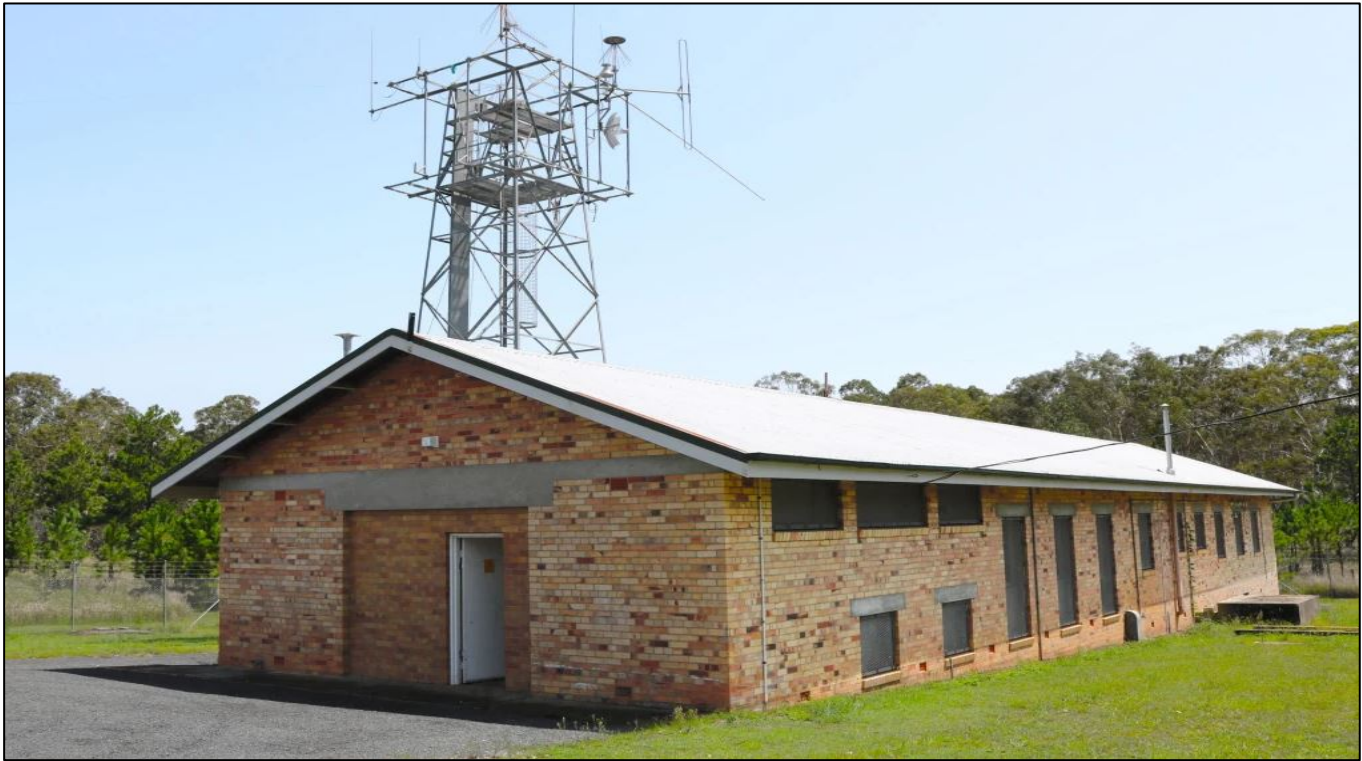
The old US Army receiving station.
