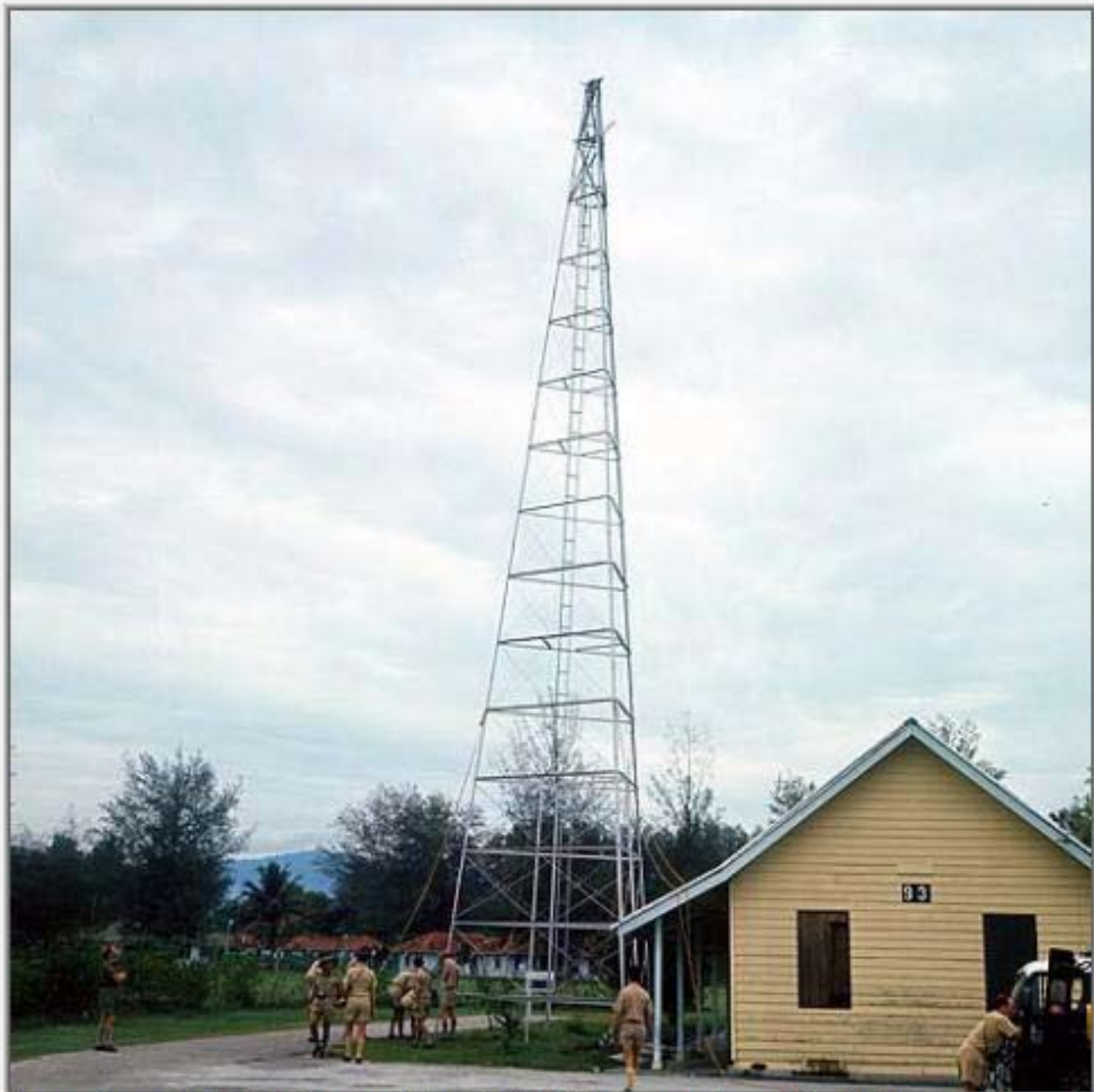
Preparing to airlift redundant Eureka/DME mast to Base Radio Transmitters site
