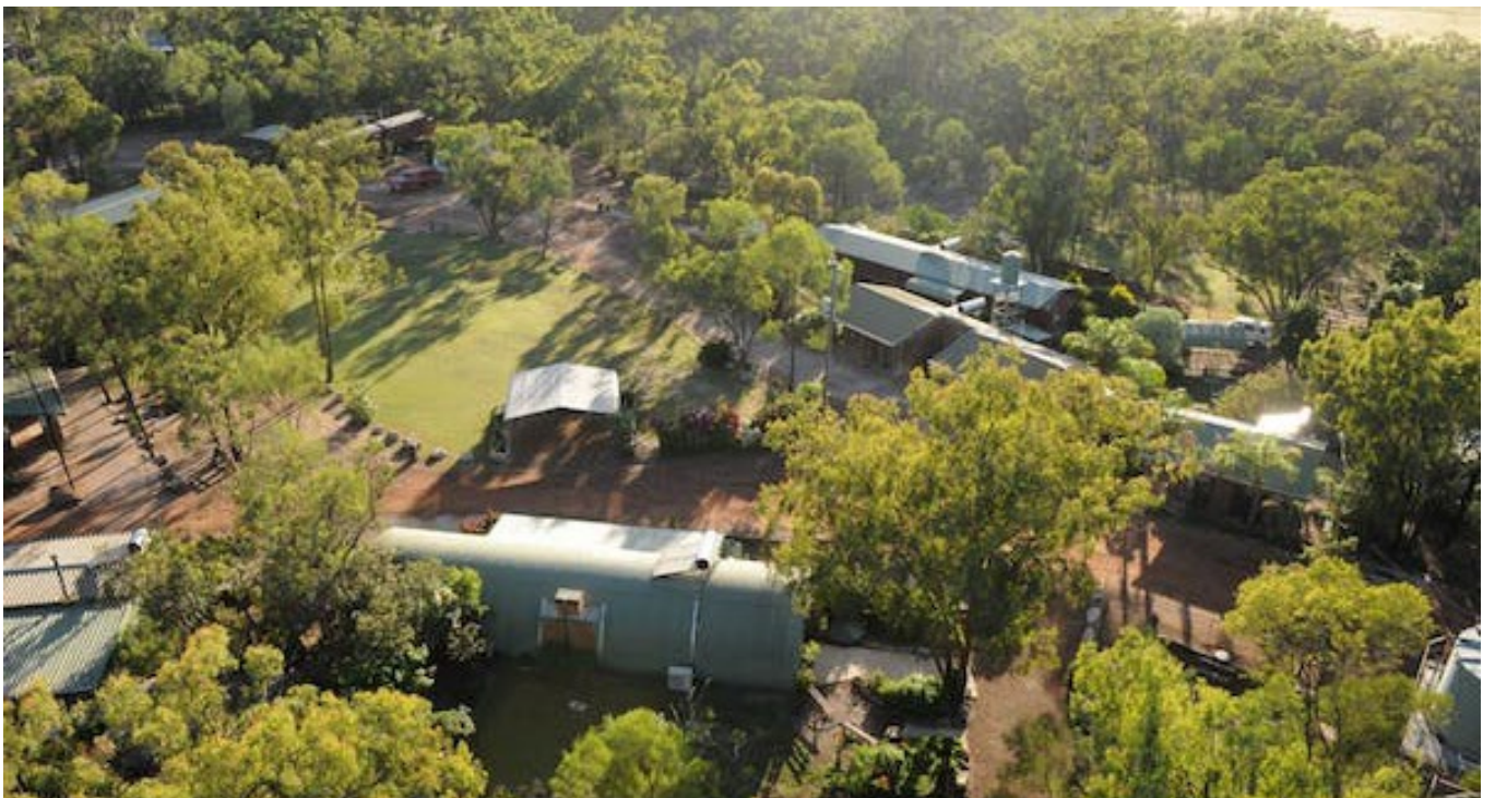
Aerial view of the complex.
