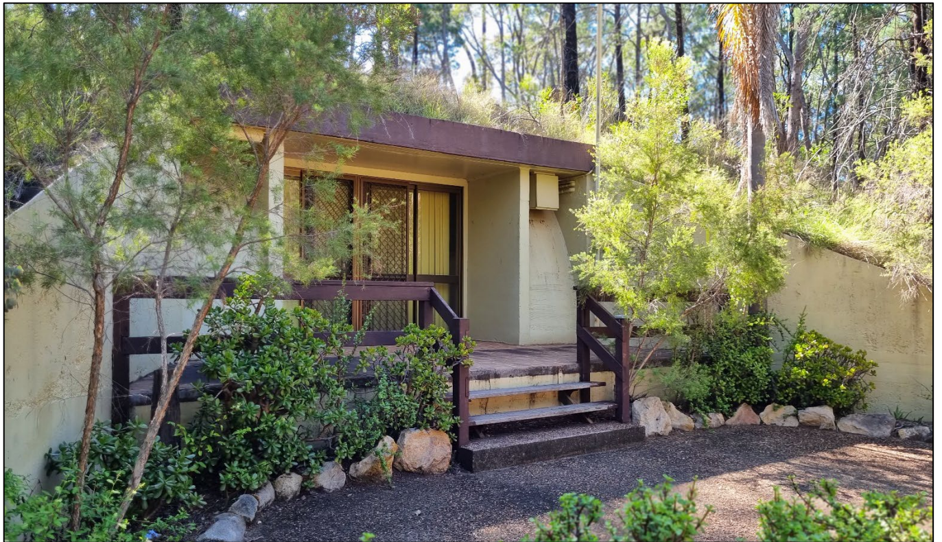
One of the refurbished bunkers.
