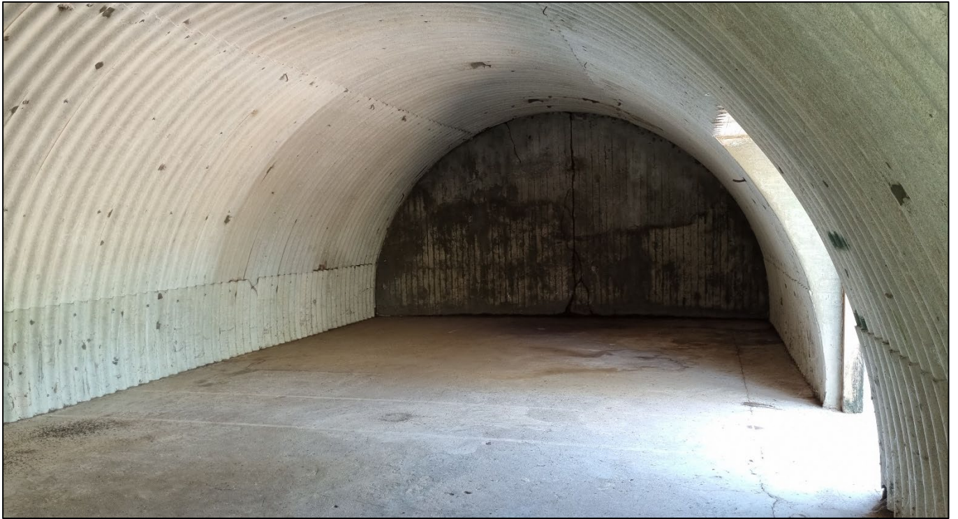
Interior of one of the, as yet, un-modified bunkers.
