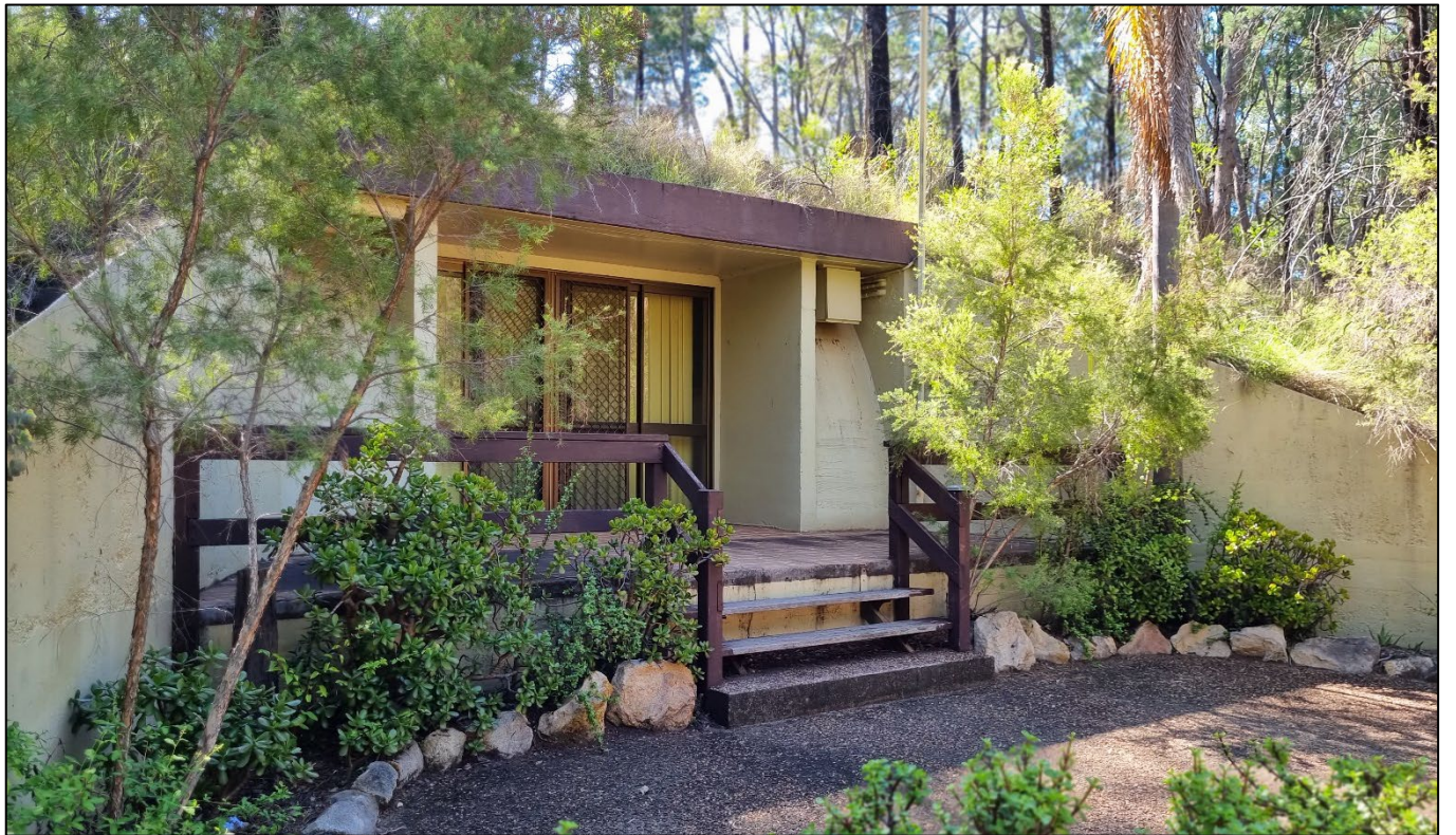
One of the refurbished bunkers.
